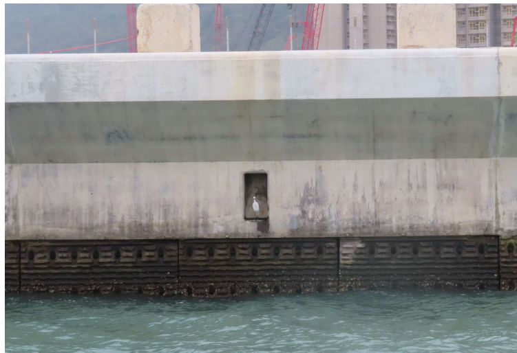
General View of Vertical Eco-shoreline
