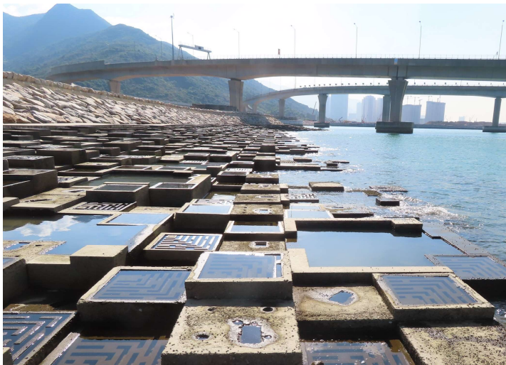
General View of Rocky Eco-shoreline
